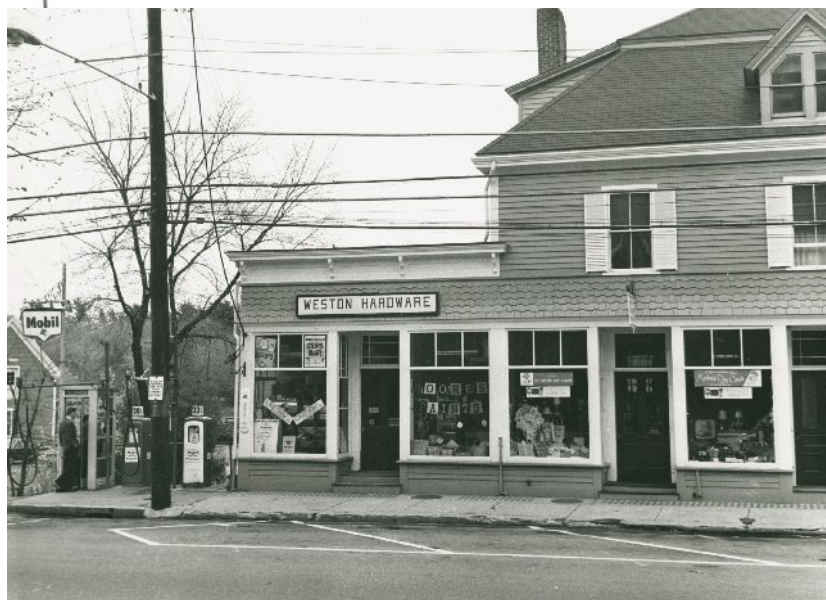
The historic preservation movement was in its infancy in 1963. The “before” photo above shows the original hardware store windows. As part of the beautification campaign, the decorative window panes were removed and replaced with the simpler window configuration seen in the “after” photo below. Notice the Mobil gas station sign, two gas pumps, and phone booth in the “after” photo. (Weston Garden Club 250th scrapbook)
