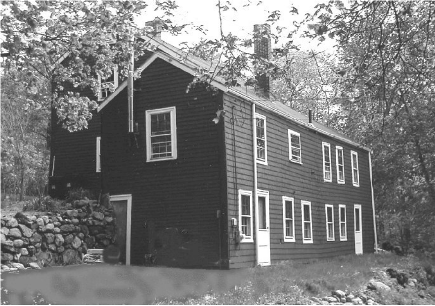
South (rear) and west facades, 2004 (Courtesy of Judy Markland)
