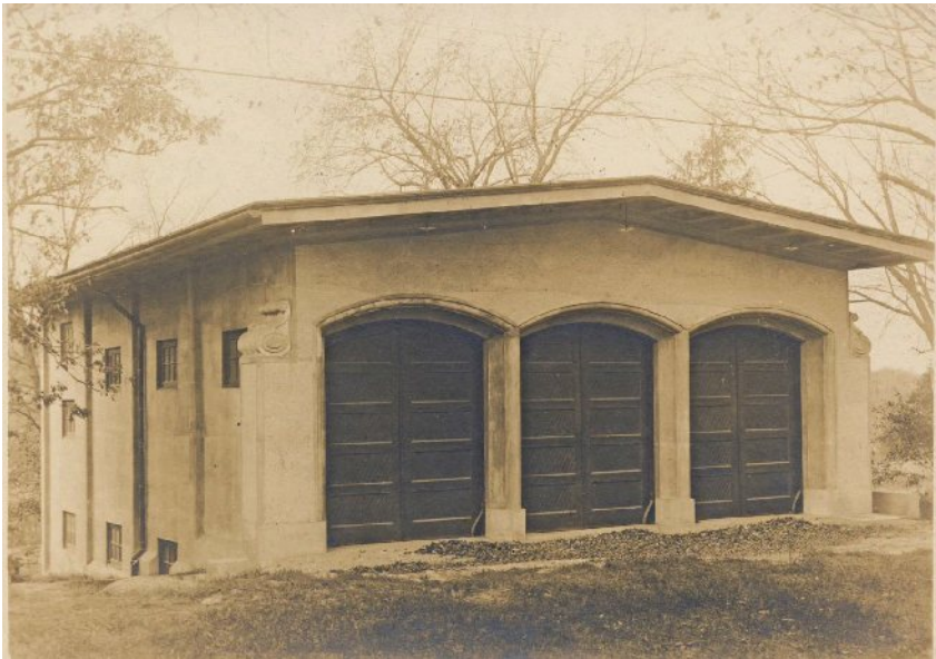
The Kendal Green fire station, was constructed one hundred years ago, in 1908. (Photo courtesy of the Weston Historical Society)
