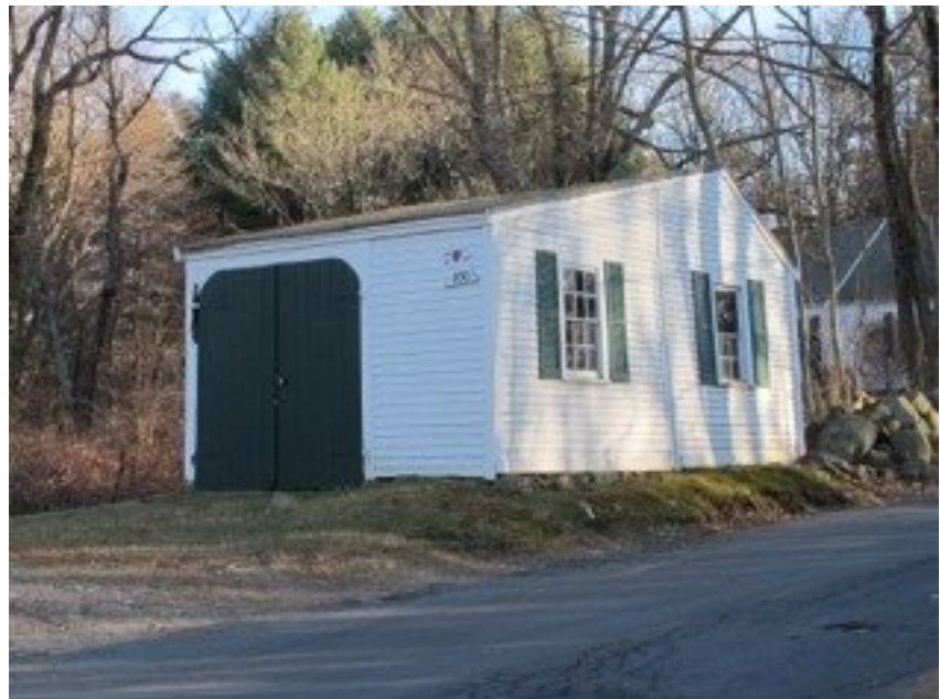
During the Depression, Oliver Patriquin moved his blacksmith shop from the town center to this small building at the corner of Love Lane and Boston Post Road. (Photo by Pamela Fox)
