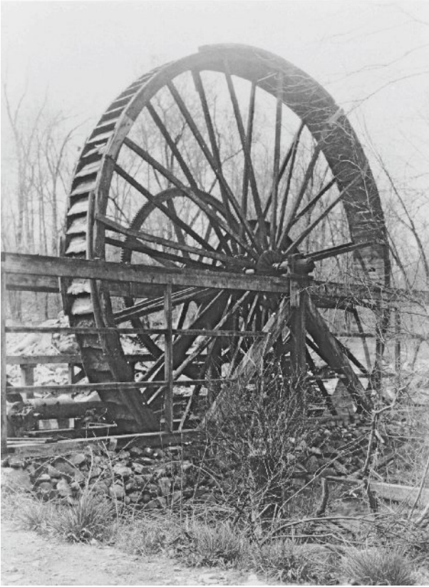
Undershot waterwheel at the school furniture factory c. 1915. Photograph by Alfred Wayland Cutting. Courtesy of Historic New England)
