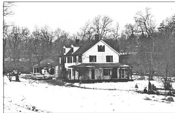
Three images of the second house on the Bush property, later numbered 92 South Avenue. (Above) Illustration from Lamson's History of the Town of Weston, showing the old Starr Farm before it was extensively remodeled by Frederick T. Bush in 1858. (Center) 1951 pencil and watercolor drawing of the house (gift of Mrs. Patricia Rice) (Below) Photograph from the mid-1950s, before the house was demolished to make way for the Massachusetts Turnpike. (Weston Historical Society photo)
