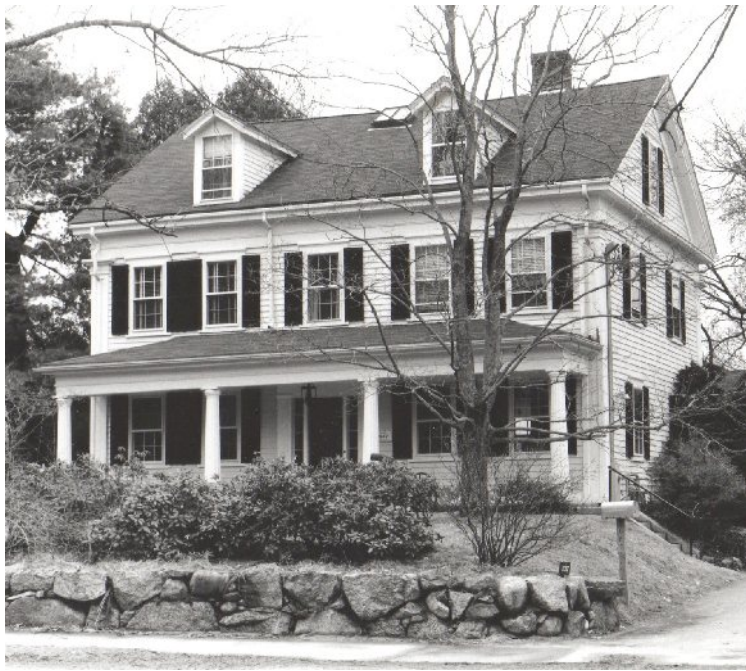
137 Wellesley Street was built for farmer Otis Train about 1847. George Milton, a Boston merchant, purchased the property in 1869 and used it as a summer place for more than 40 years before selling to Marian Case in 1912. He retained life tenancy. Following his death in 1918, the house was occupied by Theodore Chandler and his wife Mary Williams Chandler, who was a relative of Miss Case.
