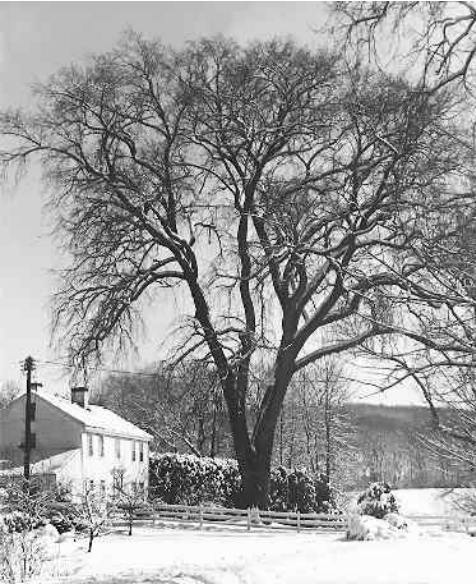
Note the size of the Colonial-era O'Toole House at 449 Old North Ave (since demolished) compared to the elm tree in front. (WHS Collection, gift of Radha Iyengar)
