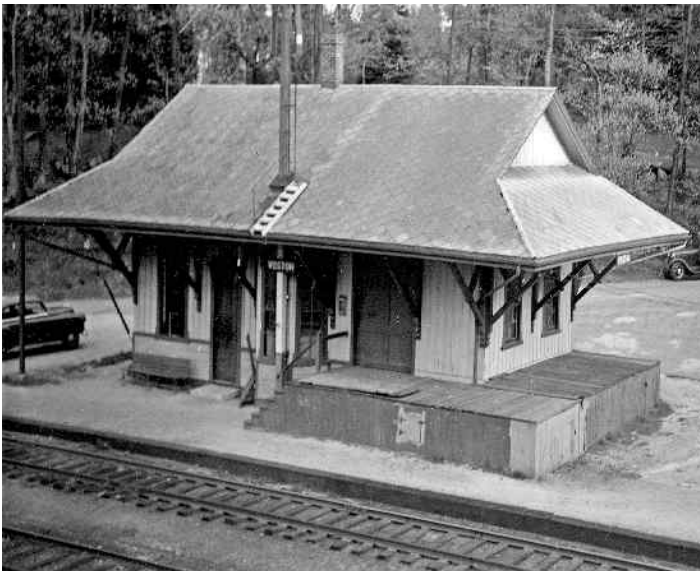
View of Weston Station in 1952 showing the gable-on-hip roof used for the important Central Mass. stations. Wayland Station has a similar roof, wide overhang, and large truss brackets. The photo also shows the main track and passing siding. (R. Richard Conard Collection)
