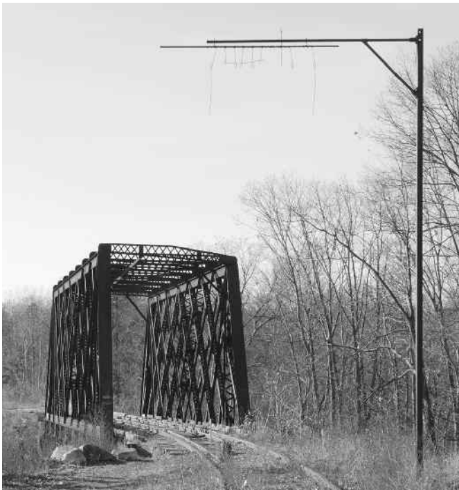
The trestle bridge and its associated tell-tale are both Treasures. This view, looking west, shows that the curve in the track extends through the narrow bridge. This unfortunate feature, a result of the original route layout in the 1870s, caused problems for railroad operations in later years. Banking the tracks to provide passenger comfort made some slow freight cars tip so much they were in danger of scraping the side of the bridge. (Photo by Valerie Mertz)
