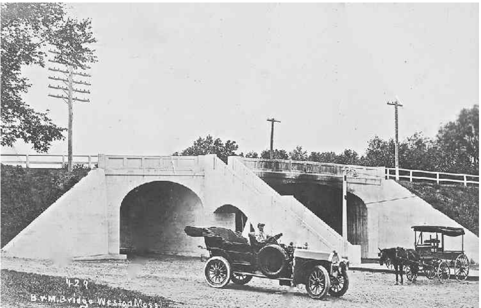
This reinforced concrete bridge was constructed in 1911-12 to eliminate the grade crossing at Church Street. The station was relocated at that time. The smaller arch allowed wagons to pass between the relocated station and the freight spur track, which remained in its original location west of Church Street. The bridge on Concord Road was constructed at the same time. Petitions were made to eliminate grade crossings on the Fitchburg line but that work was never carried out. (Weston Historical Society postcard, c. 1912)
