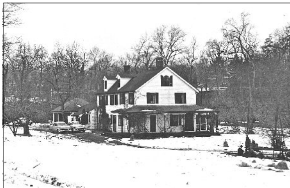
Three images of the second house on the Bush property, later numbered 92 South Avenue. (Above) Illustration from Lamson's History of the Town of Weston, showing the old Starr Farm before it was extensively remodeled by Frederick T. Bush in 1858. (Center) 1951 pencil and watercolor drawing of the house (gift of Mrs. Patricia Rice) (Below) Photograph from the mid-1950s, before the house was demolished to make way for the Massachusetts Turnpike. (Weston Historical Society photo)
