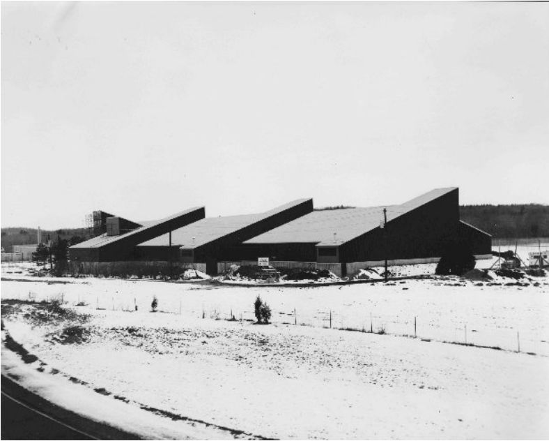
To break up the vast roof surfaces, the building was divided into three staggered sections. Note the low silhouette and sweeping lines. (Photo c.1969 courtesy Wightman Tennis Center)
