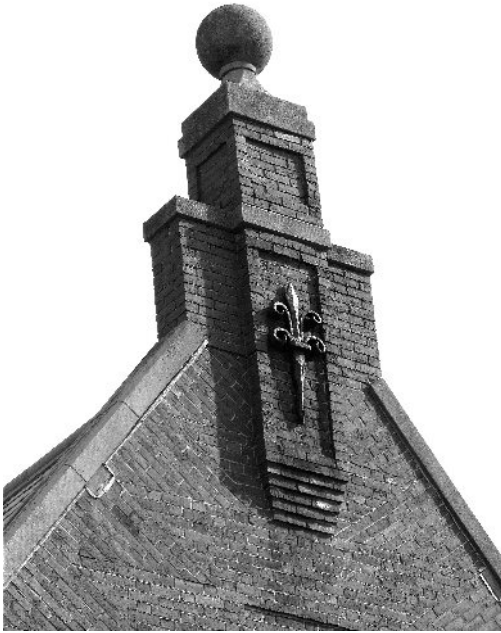
The Arts and Crafts movement emphasized the importance of materials and craftsmanship. The brickwork is particularly notable in the gable ends. (Photo by Pamela W. Fox, 2010)
