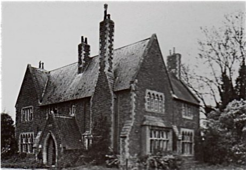
The St. Savior's vicarage in England, designed by William Butterfield and built in 1844-45, is an example of how Elizabethan and Jacobean architectural features reappeared in the 19th century, first in England and then in the United States. The kinship with Weston's 1899 library is clear, particularly in the use of brick with limestone trim to set off window groupings and door openings.
