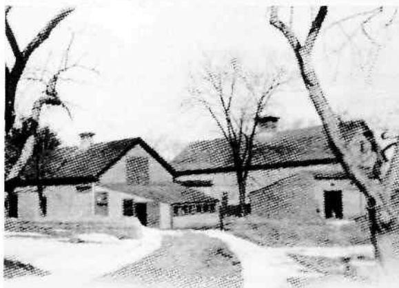
Figure 18-10. Paine built an art studio for his daughters, Helen and Georgina, who were talented painters. One side was entirely glass, to capture the north light prized by artists. Inside was a cozy fireplace under a balcony. The studio was demolished in the late 1990s. (1918 photo)
