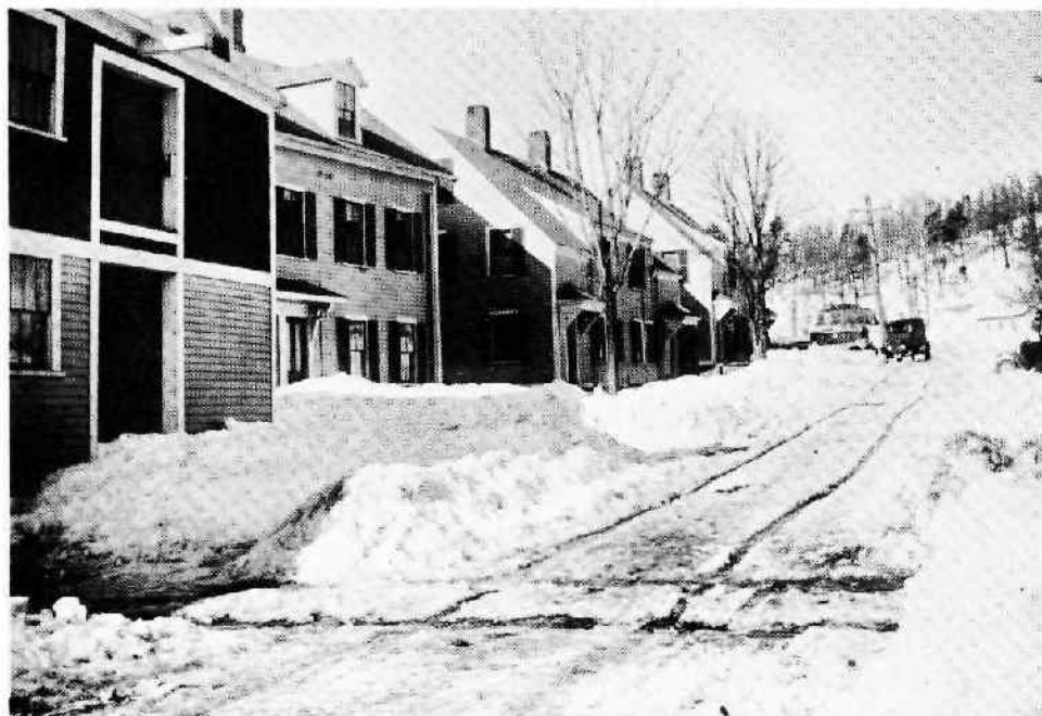
Viles Street, looking toward North Avenue, in the 1920's. At the left is the drying shed, followed by the four-tenement house razed in 1936. The last two houses, #126-134, were built in 1897 and remain in use today. Note the three automobiles in the background.
