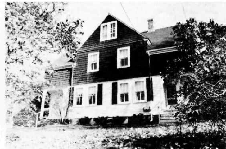
Three two family “cottages” were built in 1897 on a part of the old Warren Farm at #17-29 Lexington Street to house additional organ factory employees.
