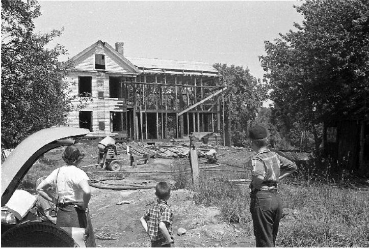
At left above and below: The Tyler farmhouse at 178 Lexington Street, during and after reconstruction in 1954. At right: 1954 photo of the Tyler farmhouse during reconstruction. (Photos by Peg Hunt, courtesy of Charles Hunt)
